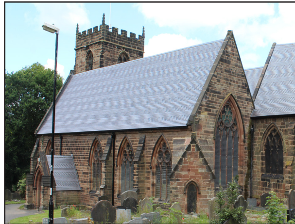
Figure 34 Street lighting within the churchyard
