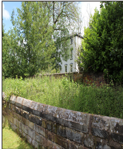
Figure 24 brick and stone walls surrounding Bushbury Hall
