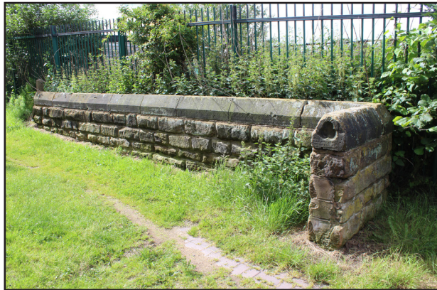
Figure 22 Stone walls of the church yard boundary
